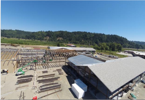
Aerial looking at Commons and west end of South Wing
