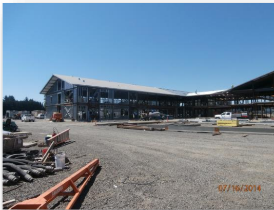
South Classroom Wing and courtyard
