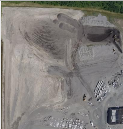
Aerial of ongoing ball field grading
