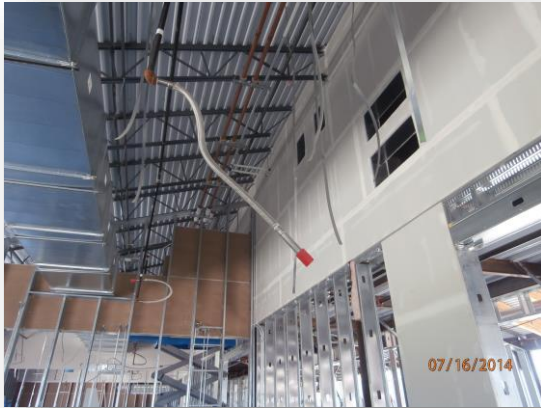
North Classroom Wing - interior
