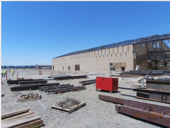
Gymnasiums with new roof framing
