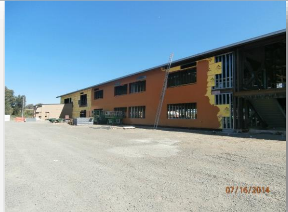
North Classroom Wing - exterior water proofing
