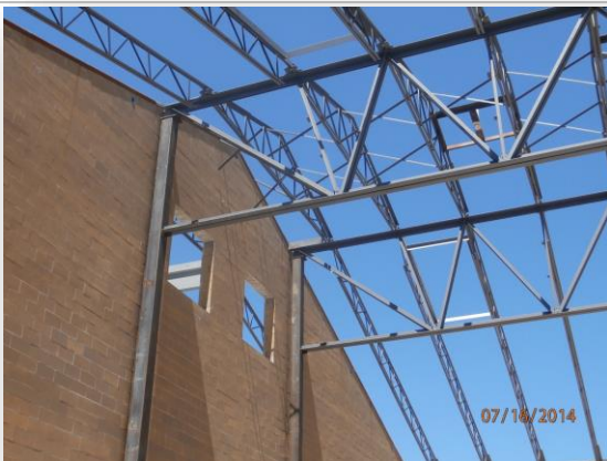
Roof framing in main Gym
