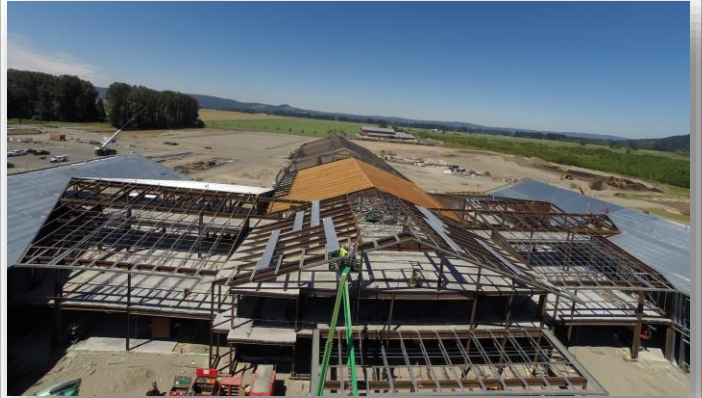
Aerial view from courtyard looking west over commons and gyms
