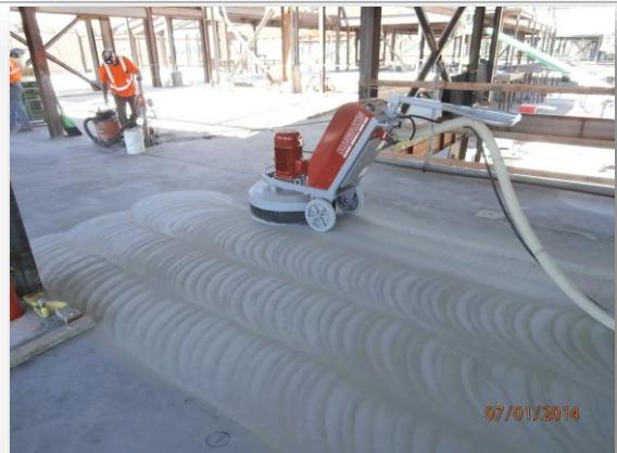
Floor polishing underway
