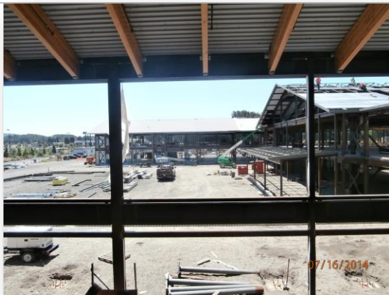
North Classroom Wing – looking into Courtyard
